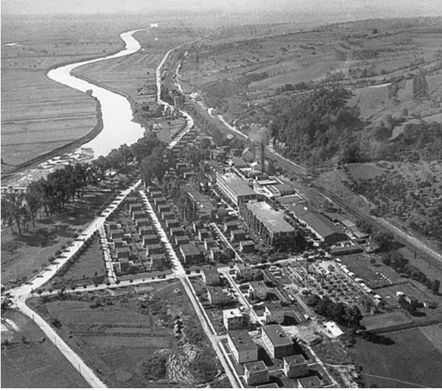
Napajedla, satellite housing estate and the Bata factory, 1936, aerial view.
