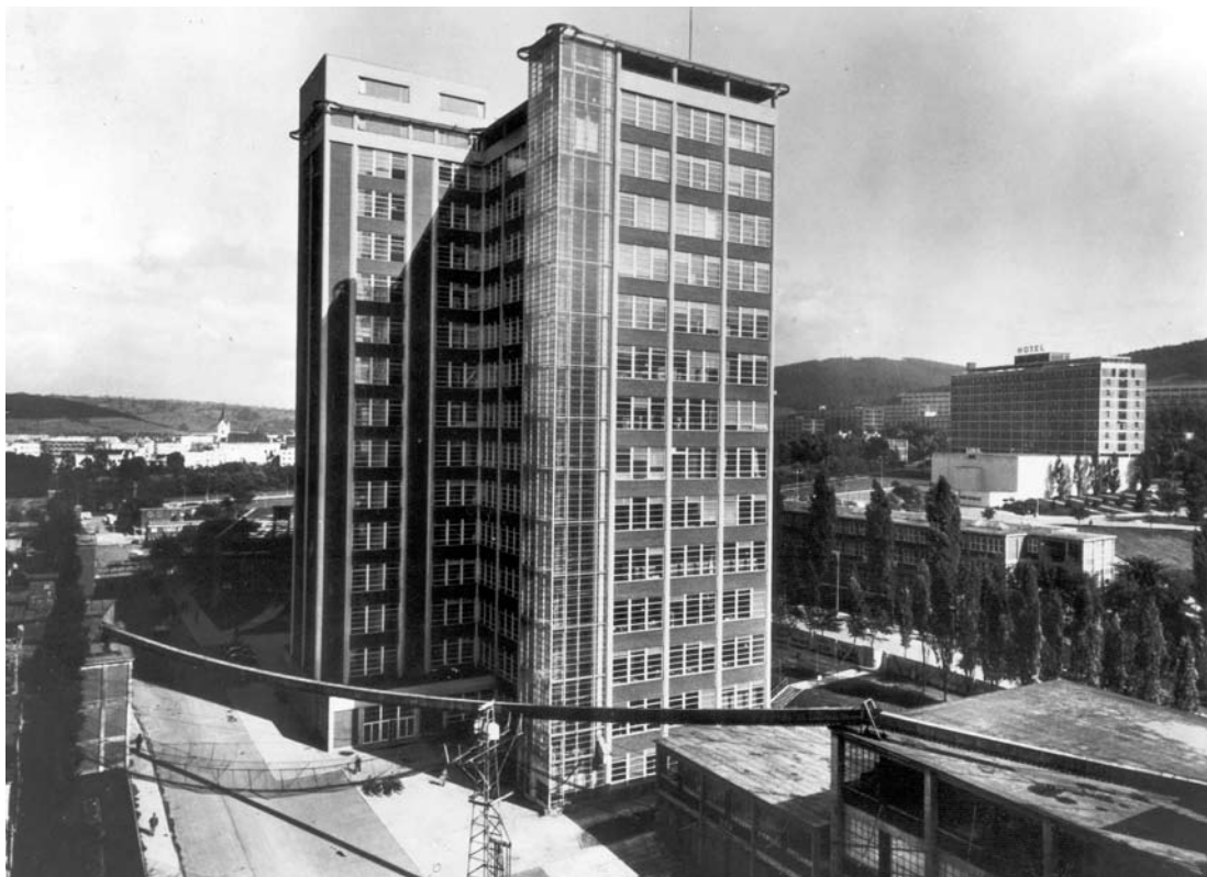
The Baťa administrative building – Building No 21, Zlín, by V. Karfík (1936-9).
