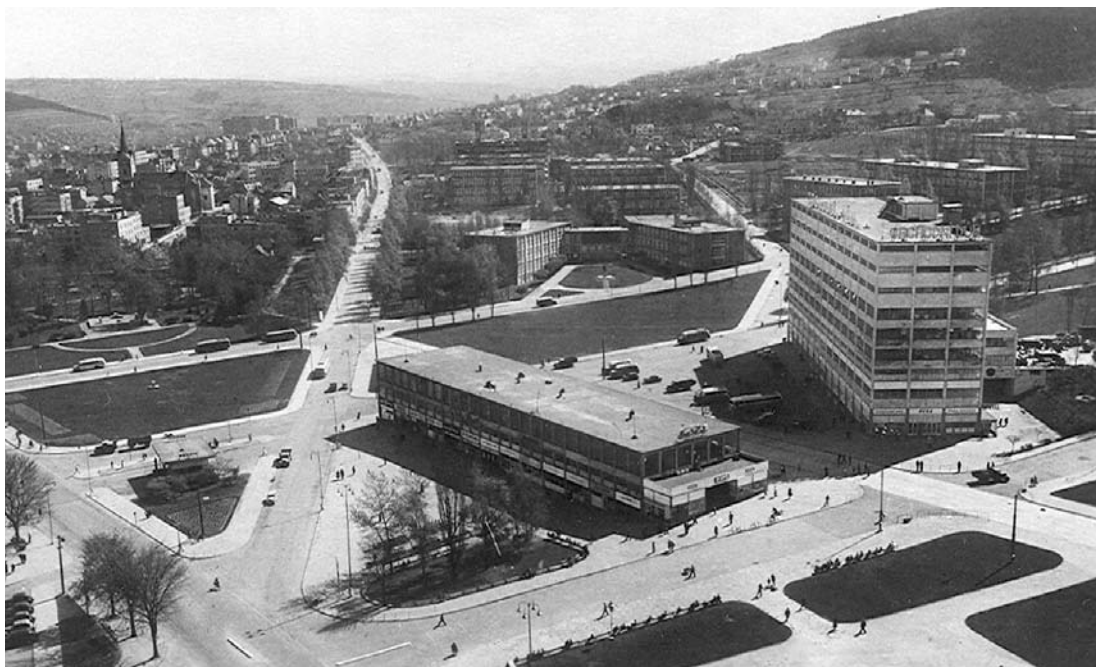
Zlín, Labour Square with the Market Hall (1928), Department Store (1929-30), and Masaryk Schools (1927) in the background.
